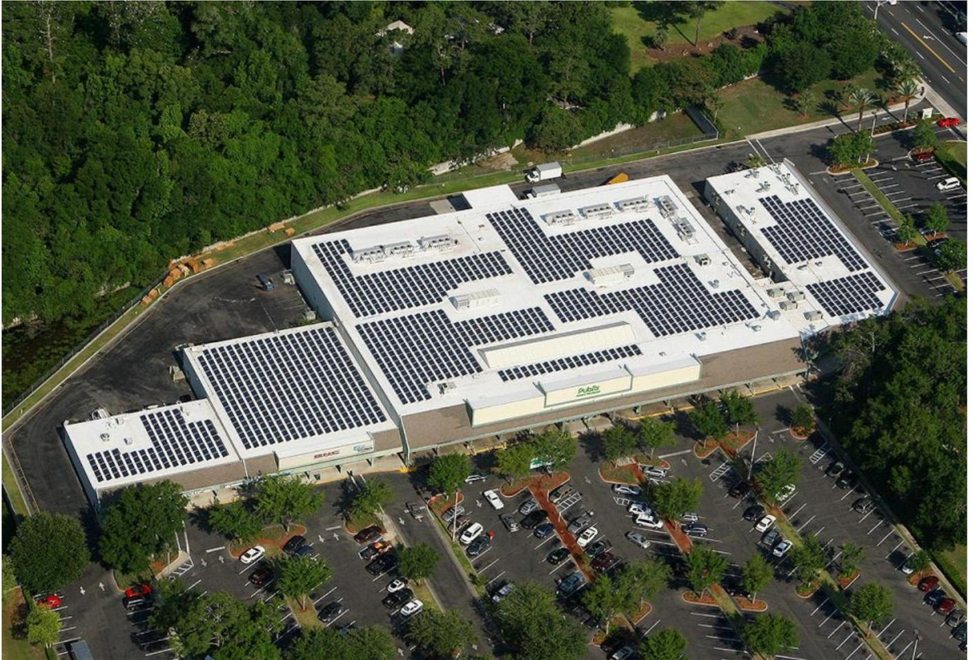
*The rooftop of a Publix-anchored shopping center in Gainesville, FL., is transformed into a 350 KW solar system populated with nearly 1,500 panels. The 46,000 square-foot installation, atop The Exchange shopping center, is among the five largest rooftop solar systems in Florida and one of the largest to use the regional utility's "feed-in tariff" renewable energy program.*
